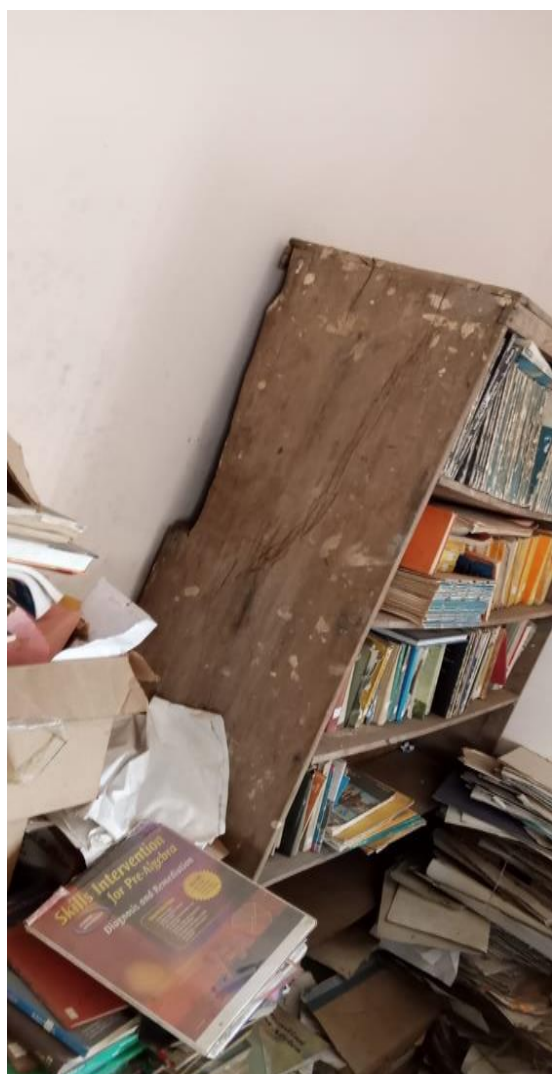
State of the Library before Renovation
